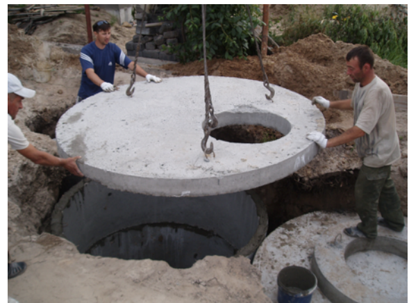
Fig. 6. Researched well during construction
